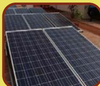
Use of Rooftop Photovoltaic solar panels with net metering facility for electricity generation-230kva
