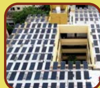
Use of Rooftop Photovoltaic solar panels with net metering facility for electricity generation-230kva
