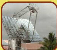
Producing steam to cook food for students through solar steam cooking system
